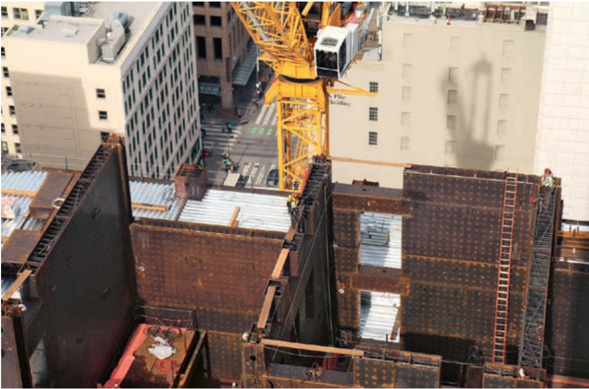
Fig. 2. The Rainier Square project in Seattle, with (left) Speed-Core panels being erected and (down) framing approaching the building's full 850-ft height.
