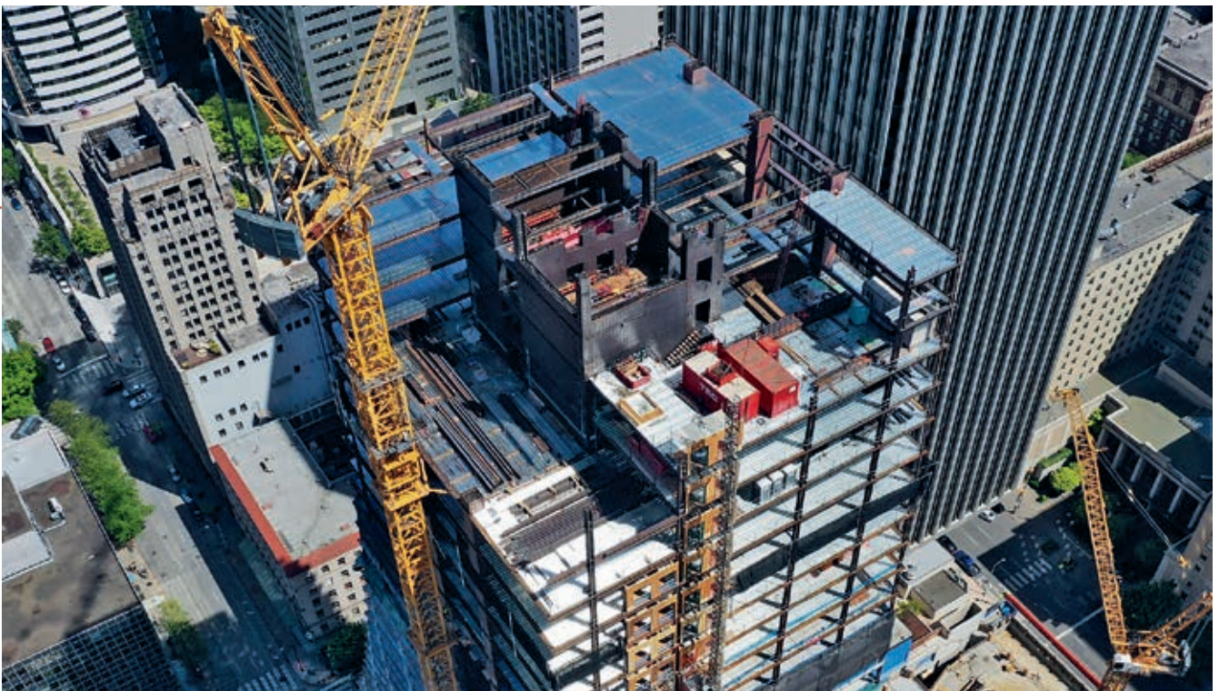
Fig. 2. The Rainier Square project in Seattle, with (left) Speed-Core panels being erected and (down) framing approaching the building's full 850-ft height.
