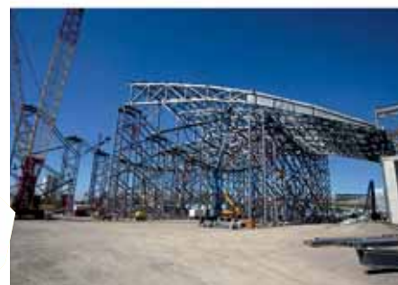
Photograph of roof erection from south support.
