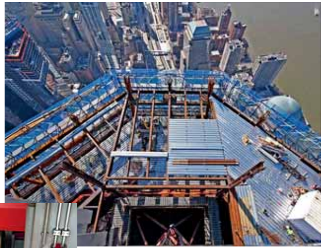
On top of the steel structure of One World Trade Center.
