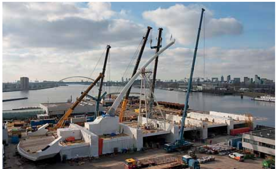
Assembly of Steel Superstructure in Rotterdam.
