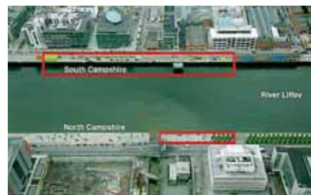
The bridge construction site area (aerial view).
