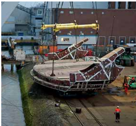
Assembly of Steel Superstructure in Rotterdam.
