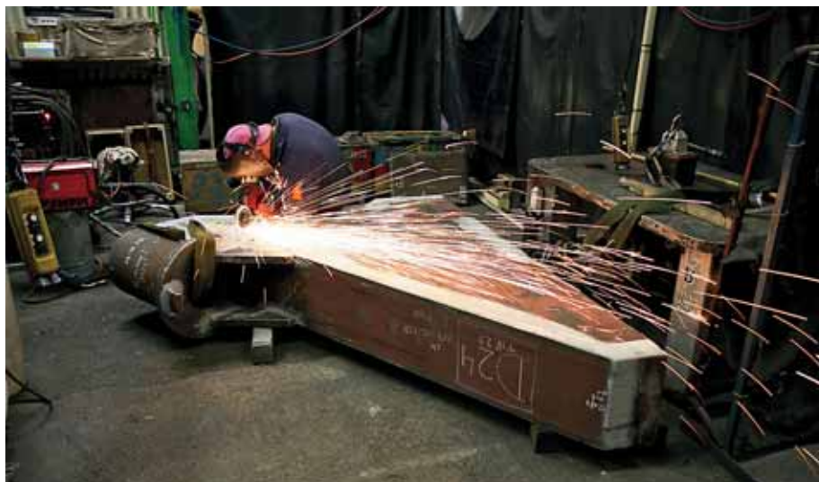
All visible welds were ground flush. Here at front anchorages.
