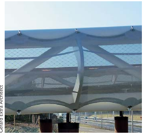
Solid wooden columns supporting the street structure covered with semi transparent fabric.
